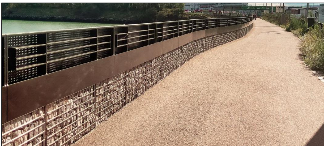
Plate 5.1 Low permeability perforated screening on the Dublin Port Greenway.
