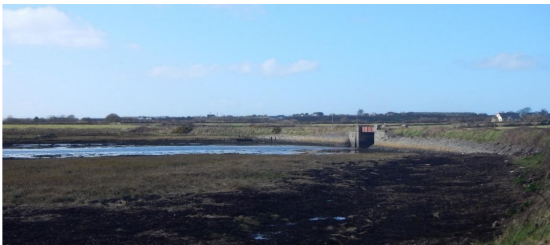
Plate 2.3 Moyasta bridge and causeway at low tide
